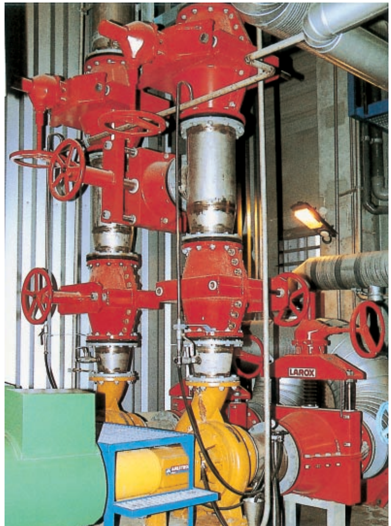
Manual valves are generally used in the pulp & paper recausticizing applications.
